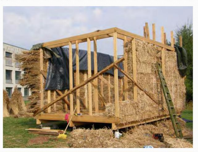
Winterizing the walls of reed house. This particular house is built on wooden framework. Bearing walls is also made of reed
